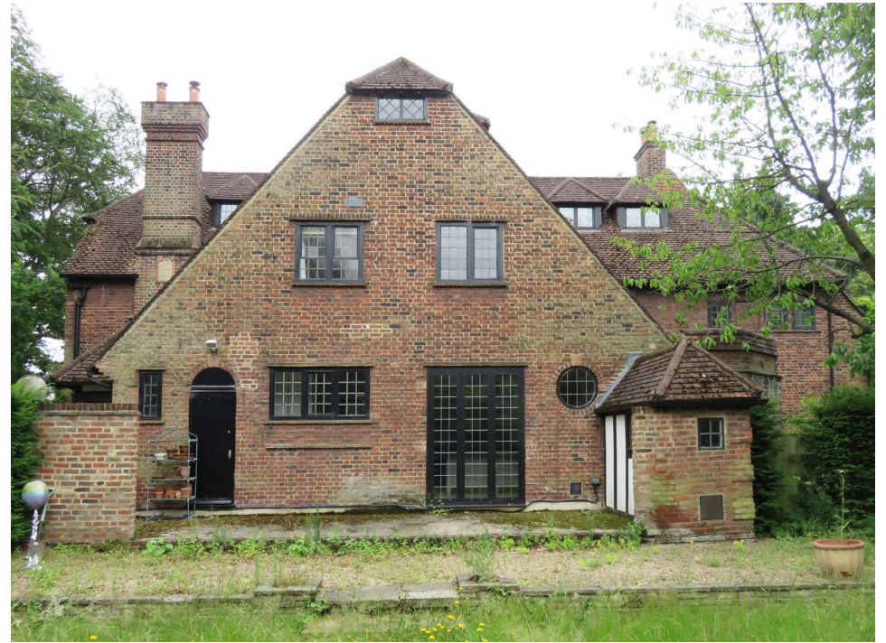
3.6 North elevation of 264 Sheen Lane, DIA 2021
