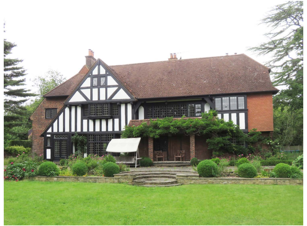
3.4 South elevation of 264 Sheen Lane, DIA 2021
