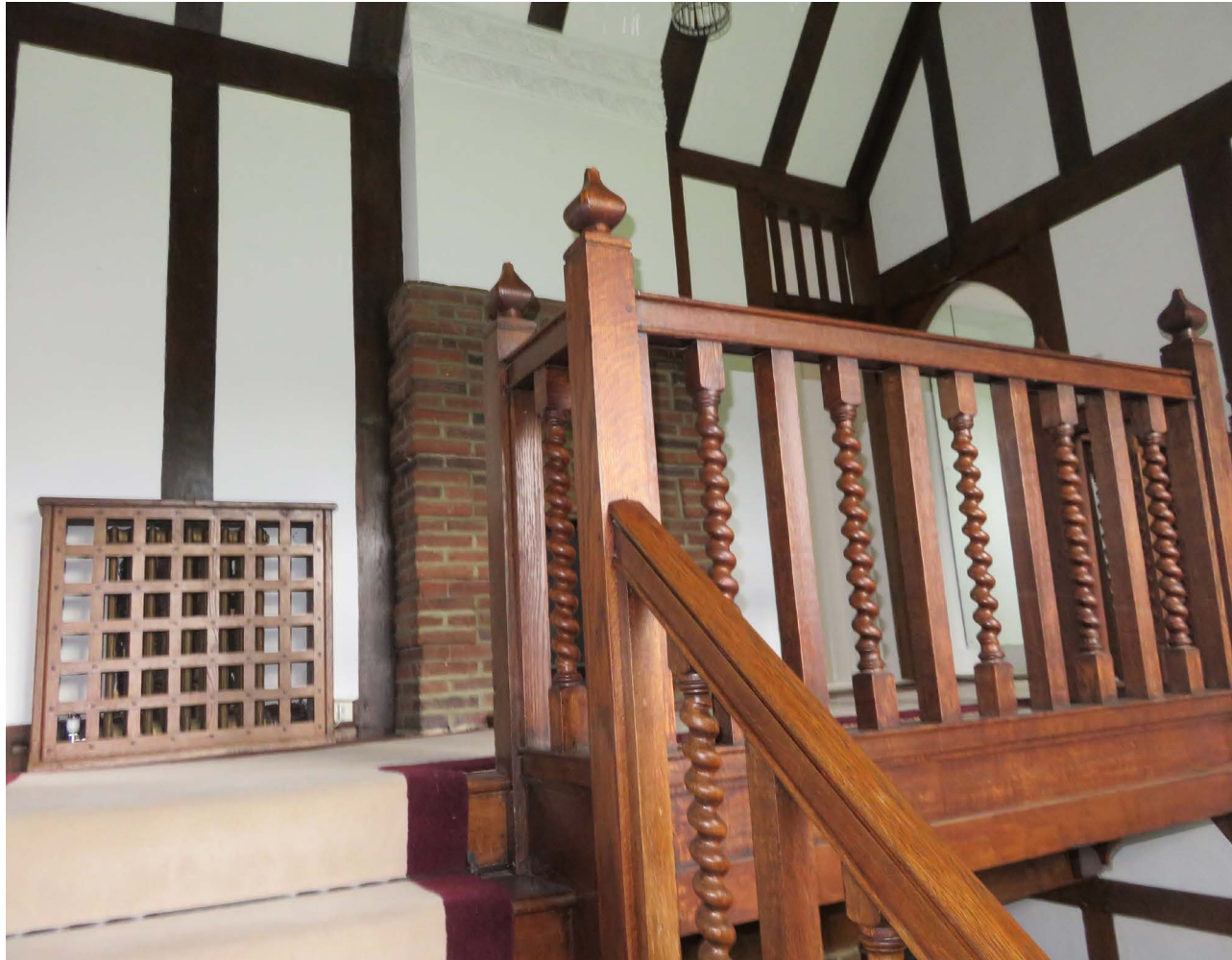
3.14 First floor gallery (F1), DIA 2021
