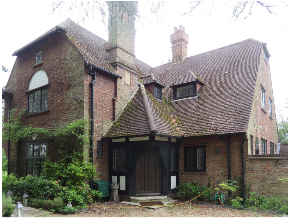
3.3 Entrance front of 264 Sheen Lane, DIA 2021
