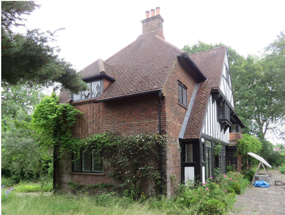
3.5 West elevation of 264 Sheen Lane, DIA 2021
