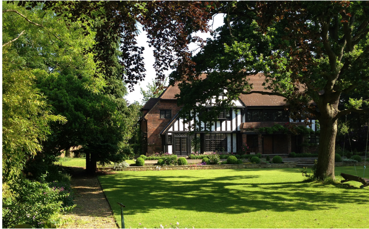
1. Sheengate view from south
