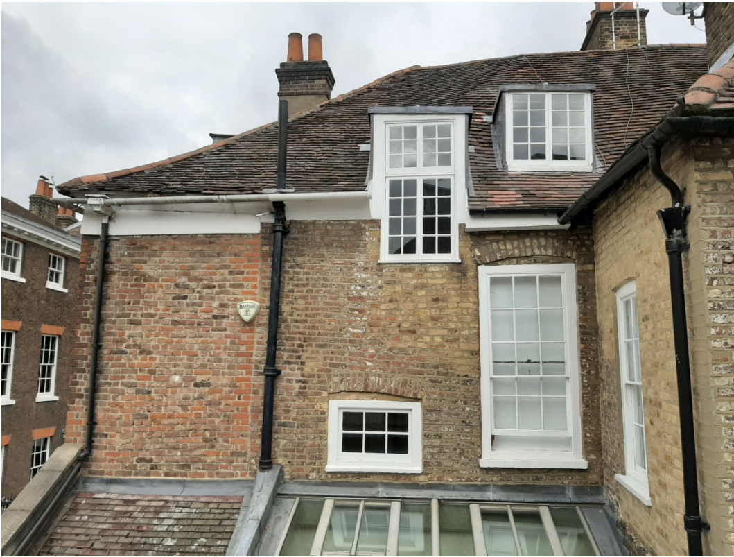
Photograph 03 – View from rear of 19a King Street
