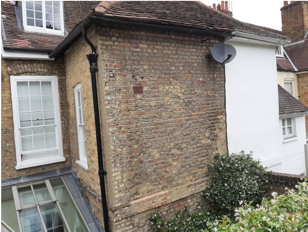
Photograph 04 - View from rear of 19a King Street
