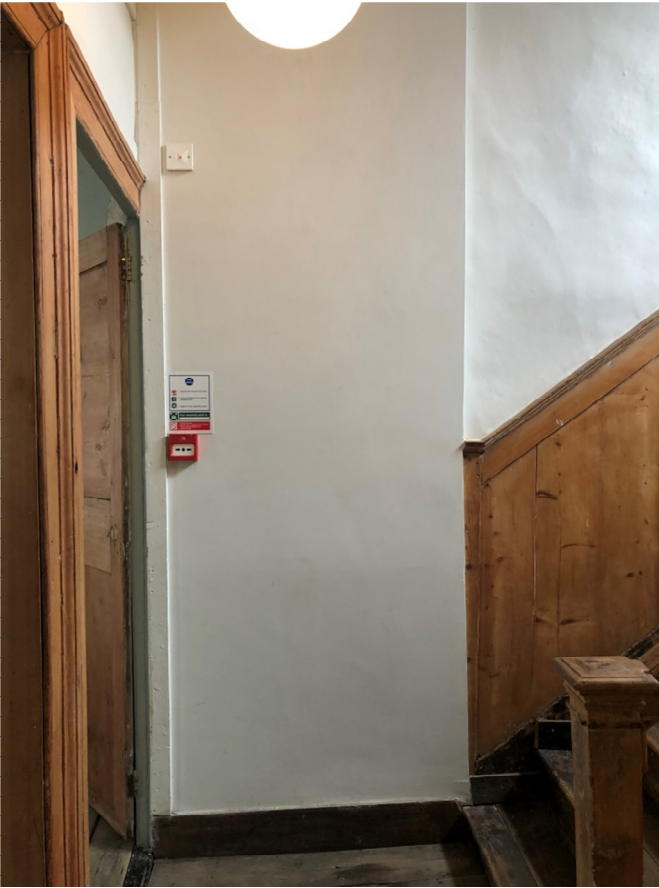
Photograph 09 – Staircase in no.19
