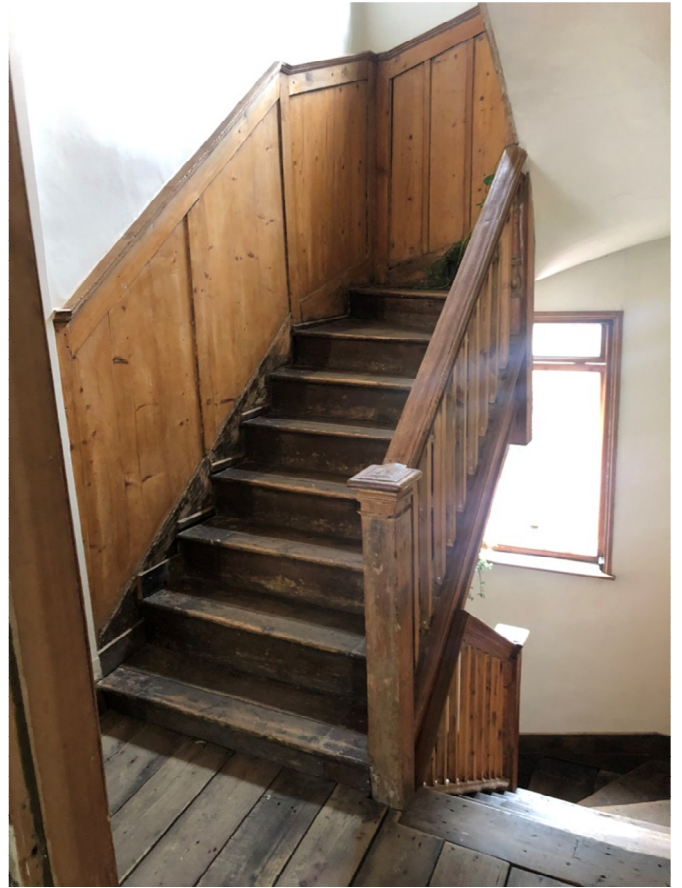
Photograph 10 - Staircase in no.19
