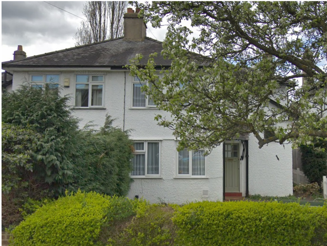
No.31 Kings Road, pre-works (Google Streetview, April 2018)
