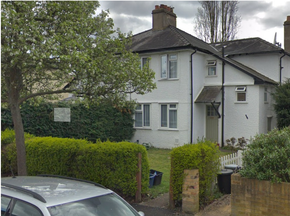
No.31 Kings Road, pre-works (Google Streetview, April 2018)
