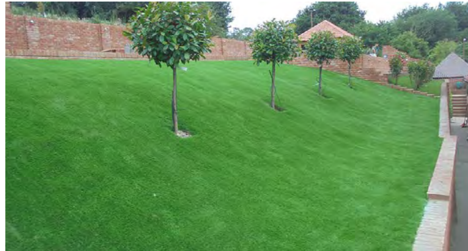
Recycled bricks - raised kerbs and retaining wall
