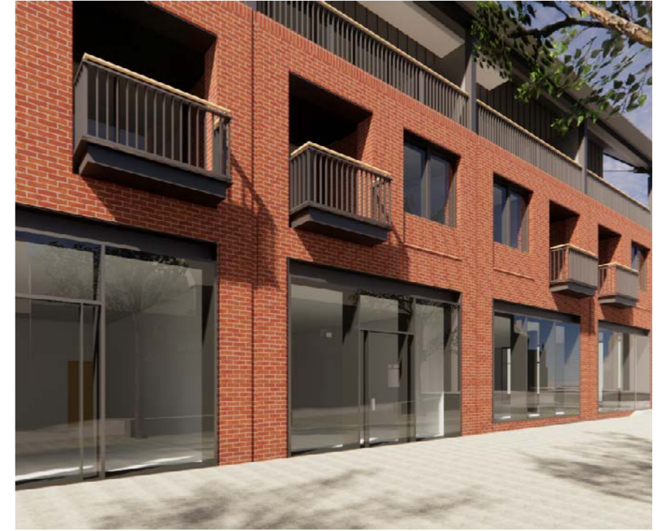
The retail units have been widened by removing every other brick pier
