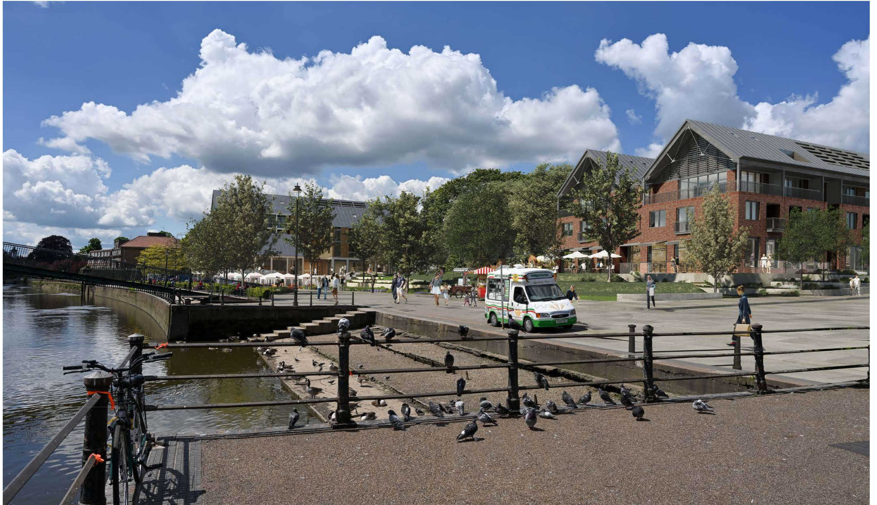
View looking back at the Water Lane building's river facing gable end
