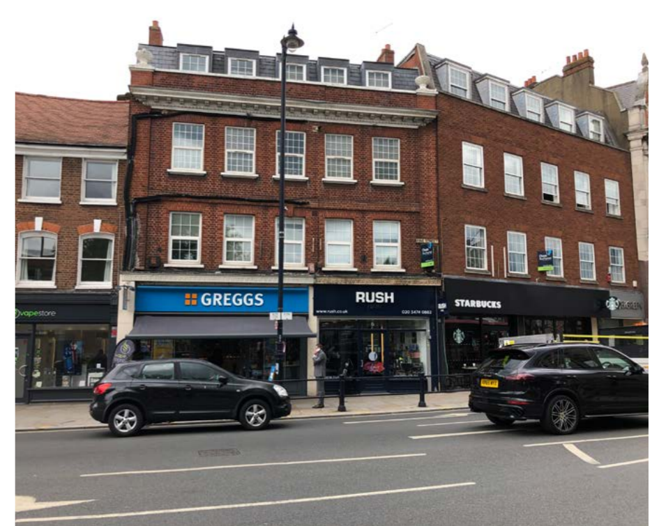
...but the buildings on the other side of the street are higher with significant changes in height
