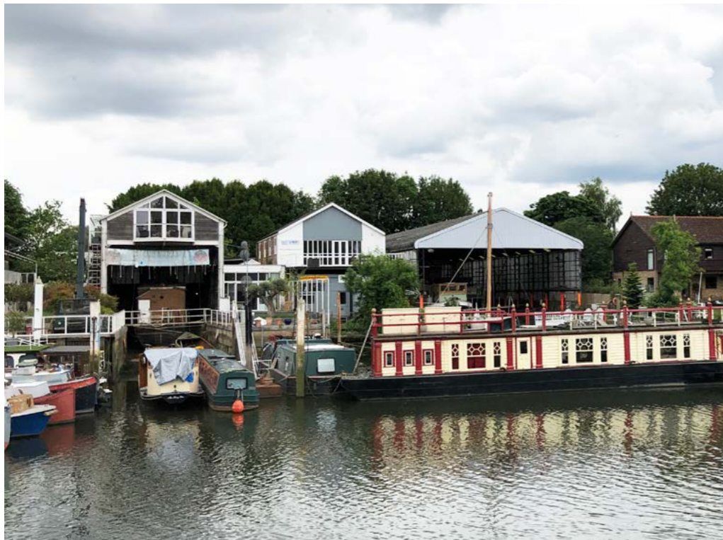
River context - steel framed boatyards on Eel Pie Island
