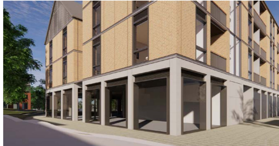
Ventilation recesses above the office windows
