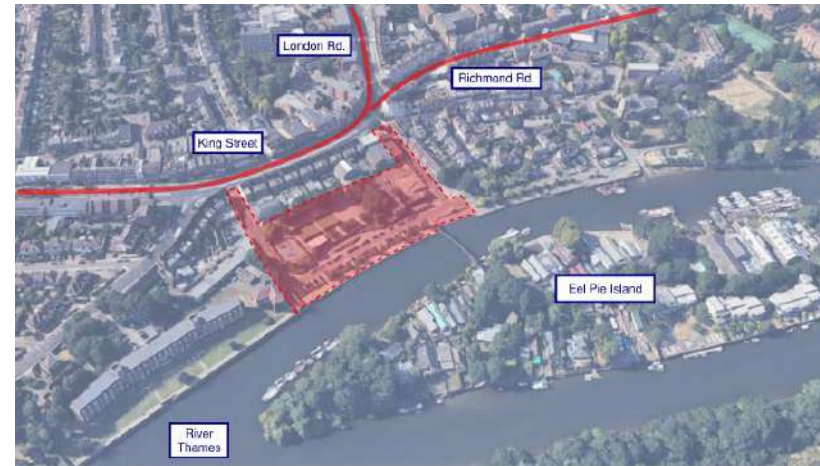
Figure 1: the Site aerial view and local points of interest
