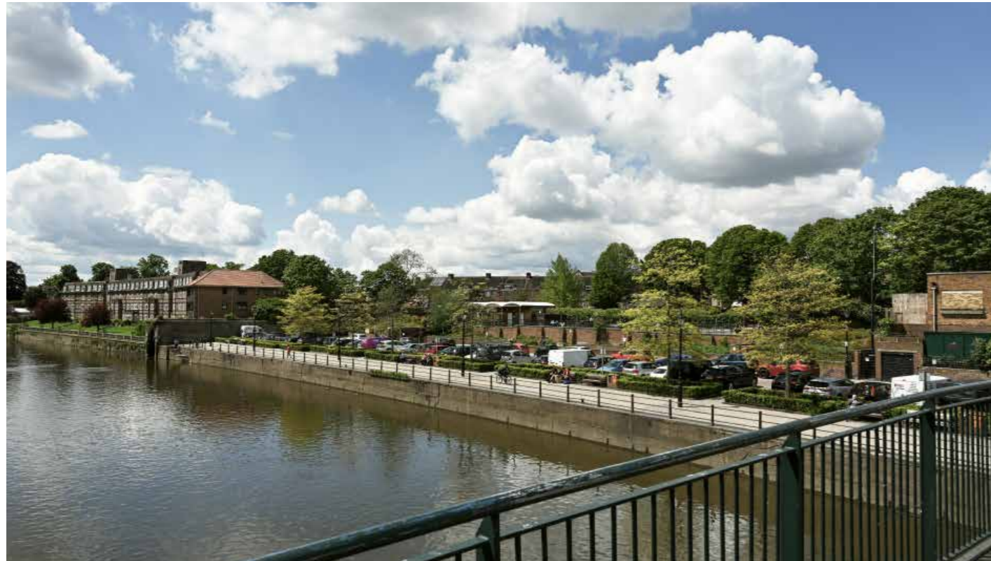
View 3A: Looking north-west from Eel Pie Island - pedestrian bridge
