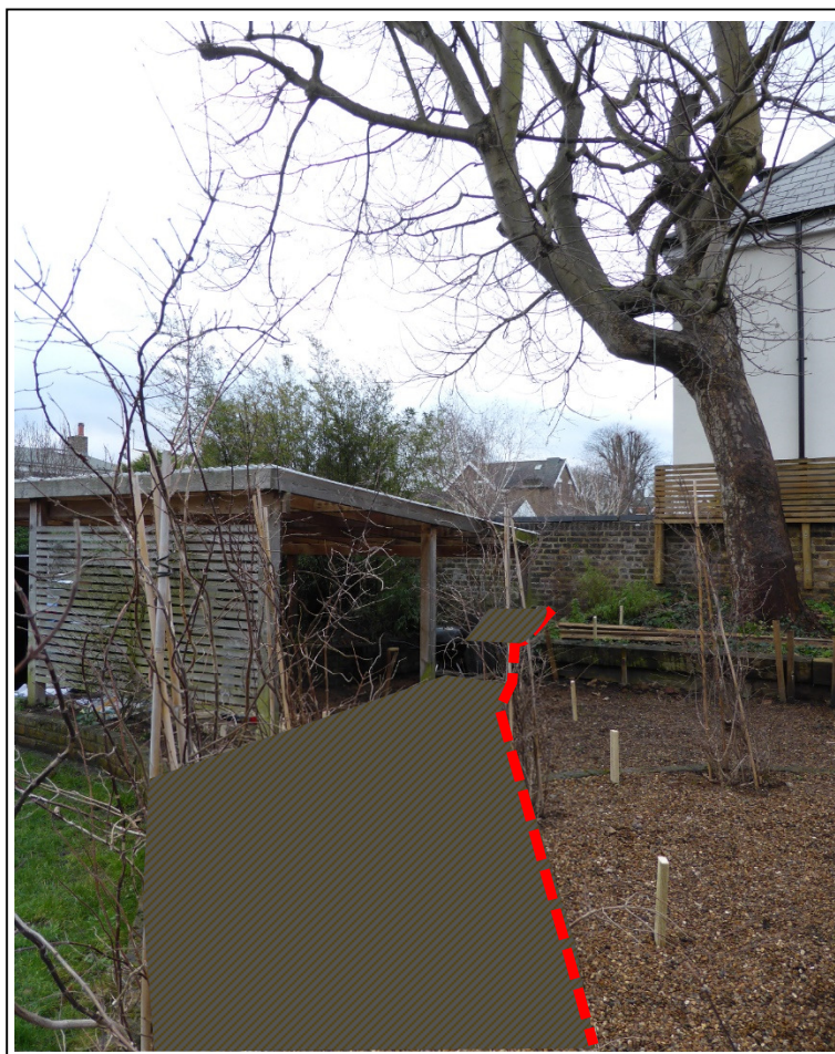
Photo 1: Location of TPB and temporary ground protection as marked out on site
