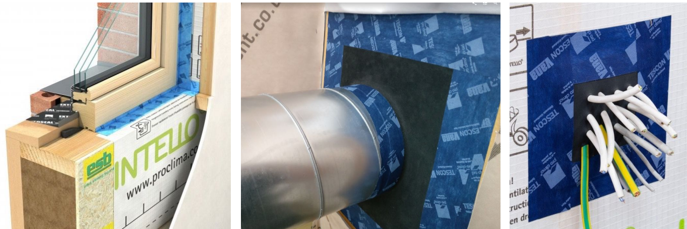
Example window reveal, MVHR duct and incoming cable penetrations through an airtight zone.
