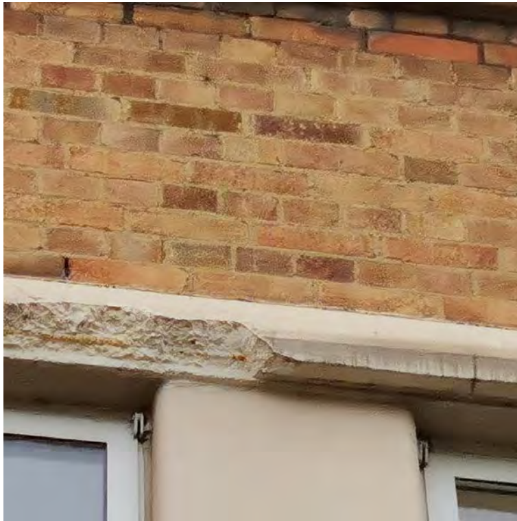
Photograph 15 – Weep holes on B3
