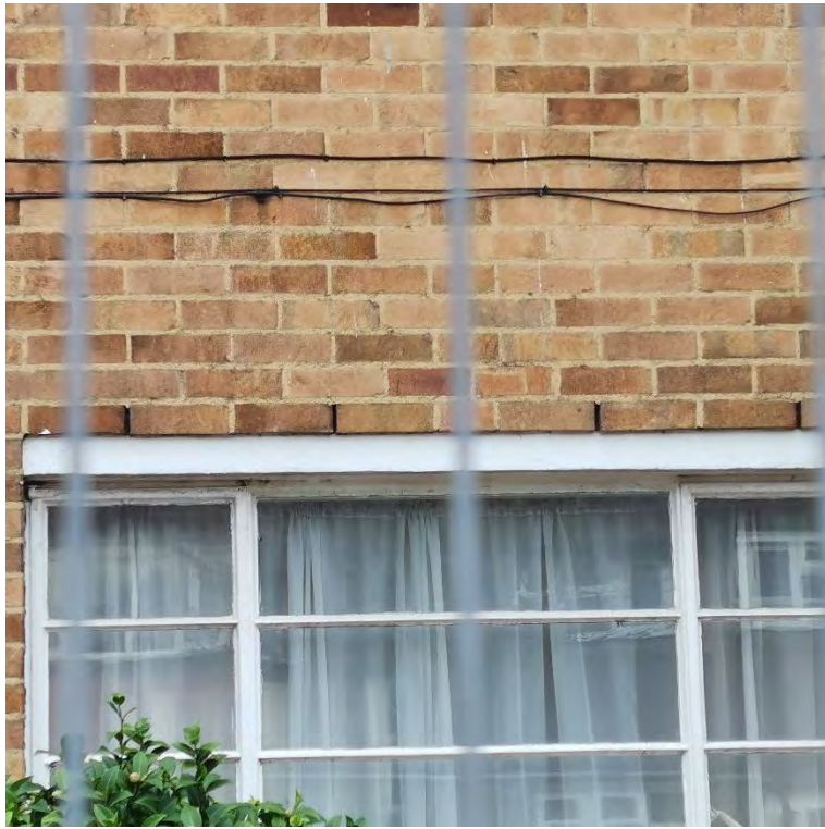
Photograph 21 – Weep holes above window on B5
