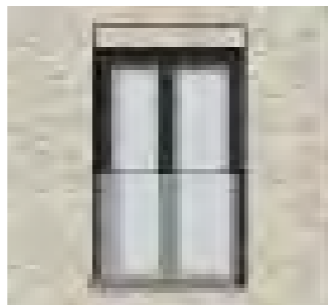
Description Double Window Pane with Glass Juliet Location Houses
