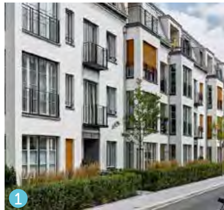
1 Private gardens with evergreen hedges and metal railing boundary treatments
