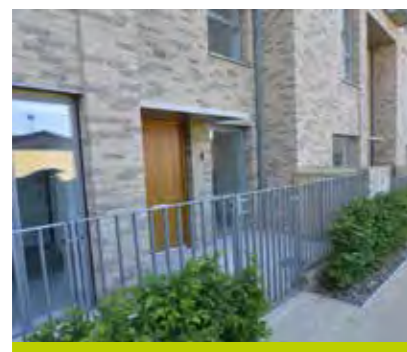
Boundary type 1 - Front gardens Metal railing with powder-coated finish, to match architecture (1.1m height)
