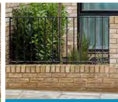
Boundary type 3 - Front gardens Brick wall topped with powder-coated metal railing, brick and railing to match architecture (1.1m height)
