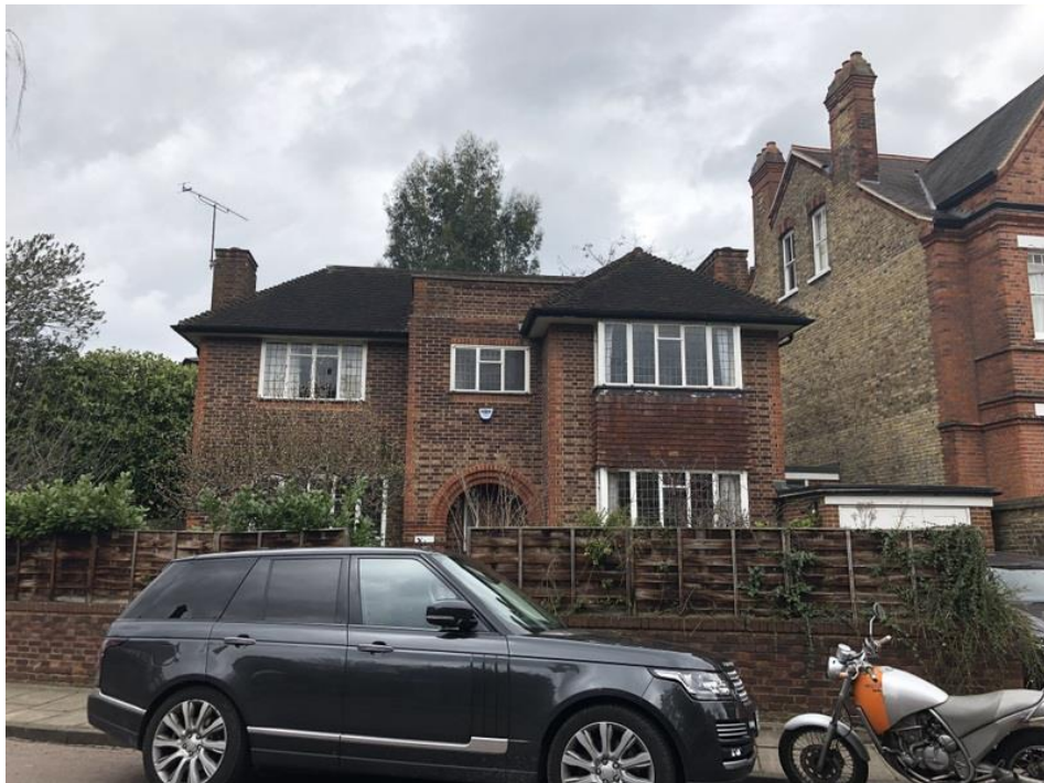
Figure 1: Front elevation of 25 St George's Road, the application site
