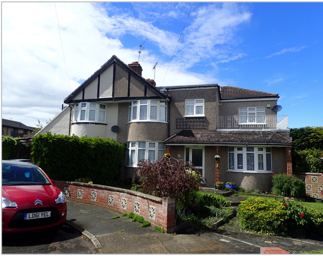
Photo 1 - 38-40 Vincam Close - front elevations
