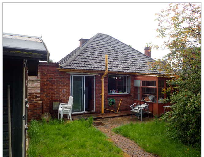
Photo 6 - 42 Vincam Close back garden area
