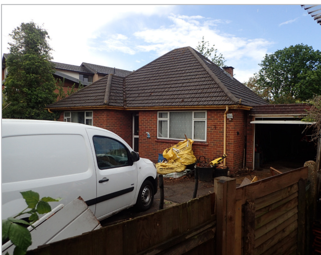
Photo 5 - 42 Vincam Close front elevation
