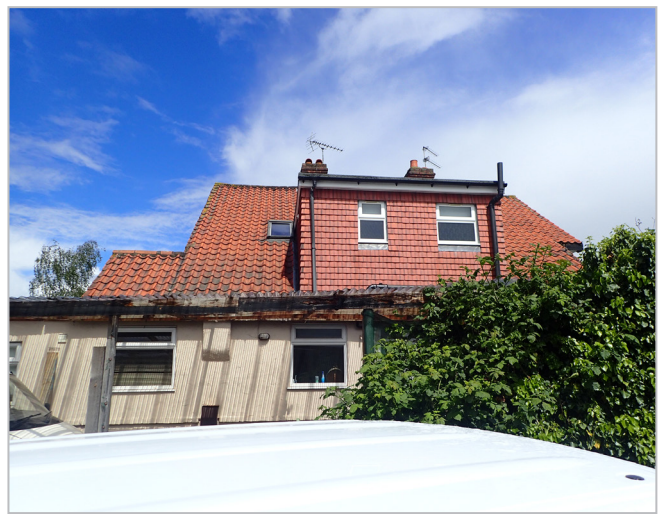
Photo 4 - 40 Vincam Close side elevation
