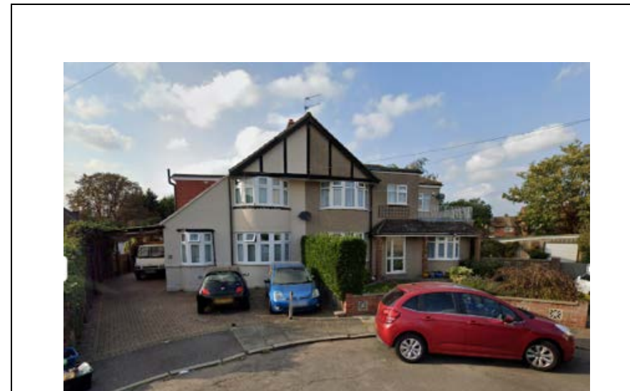
Figure 2: Existing Dwelling Photos 38 and 40
