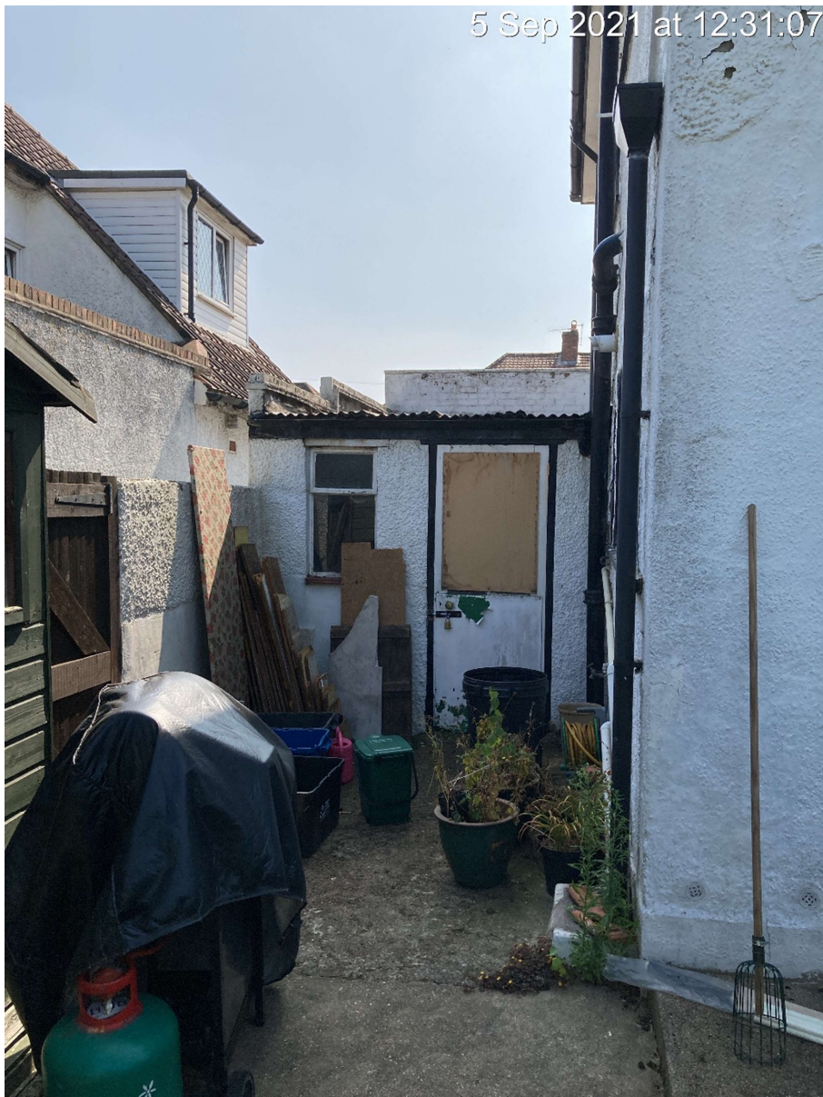
Facing the rear of 75 Cypress Avenue, showing rear of garage and gate to shared passage with No. 77
