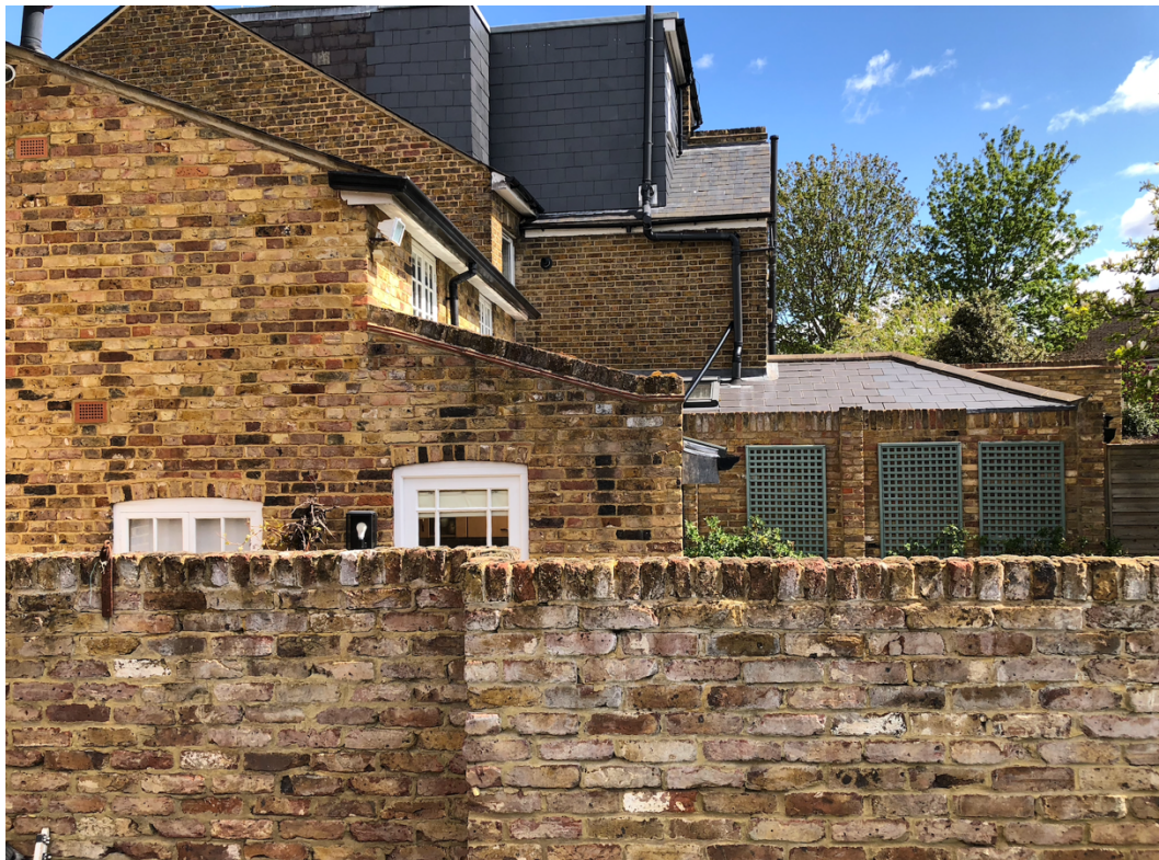
Fig 4 Adjoining development at n° 13 & 11 Middle Lane
