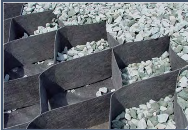
Figure 10 Examples of Cellweb filling with angular stone
