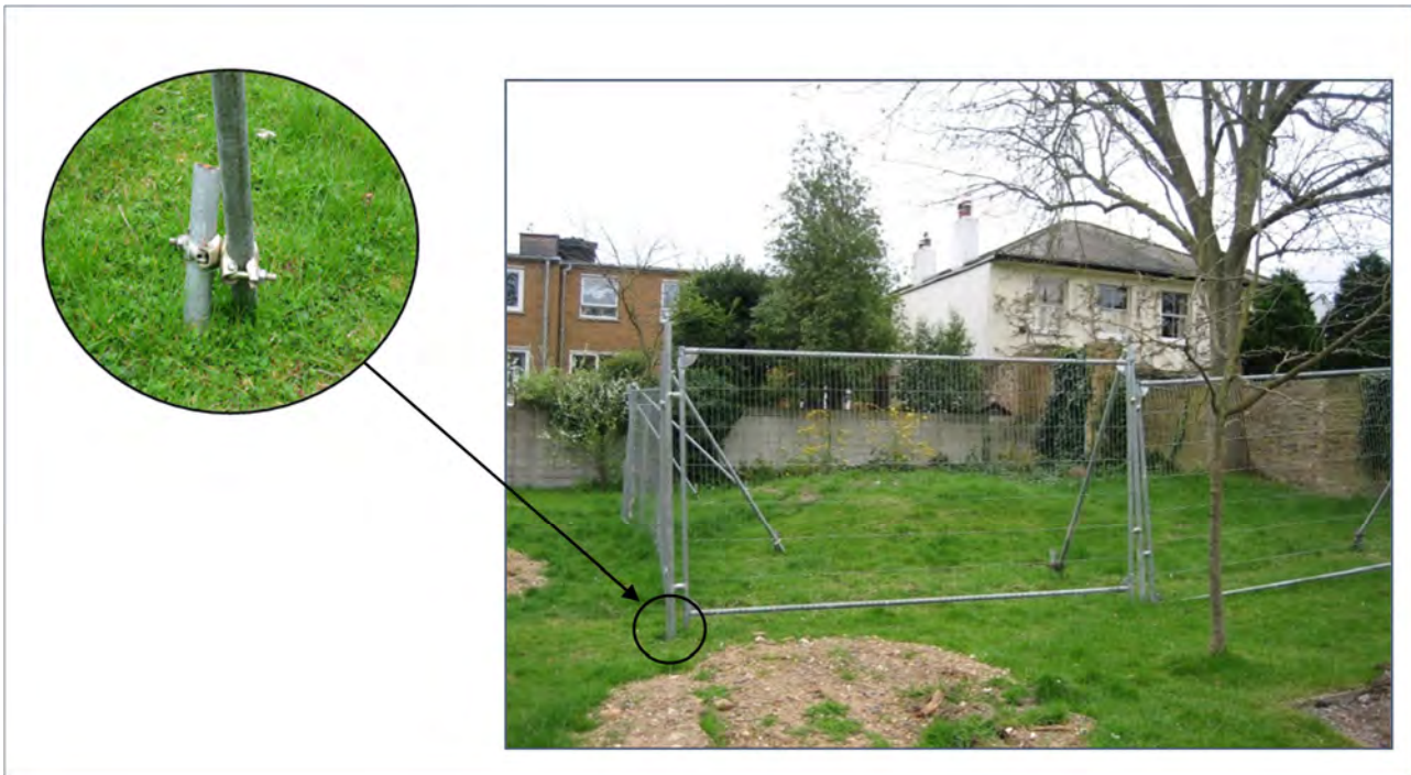
Figure 2 Example of welded mesh barriers in use
