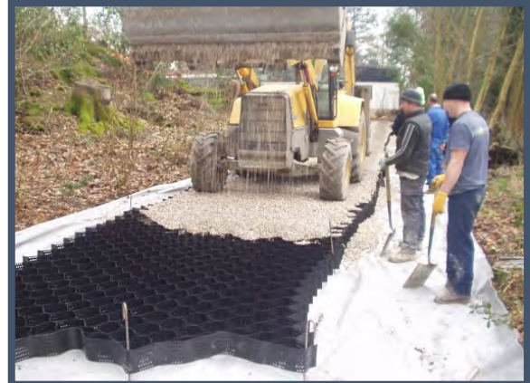
Figure 10 Examples of Cellweb filling with angular stone
