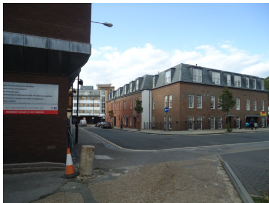
View from Castle Yard towards the extended former Police Station
