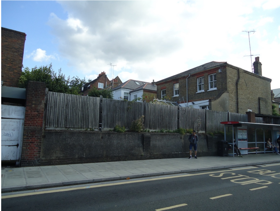
Rear and north-west flank Fairlawn, seen beyond the rendered retaining wall and timber boarded fence of the rear garden
