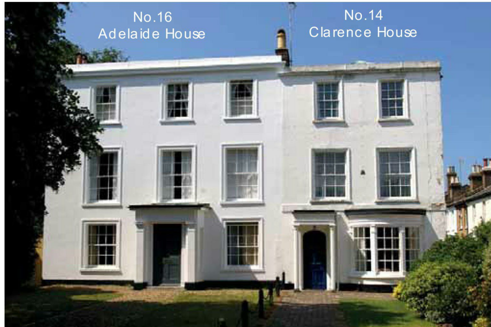
Adelaide House, 16 Park Road/ (Left)
