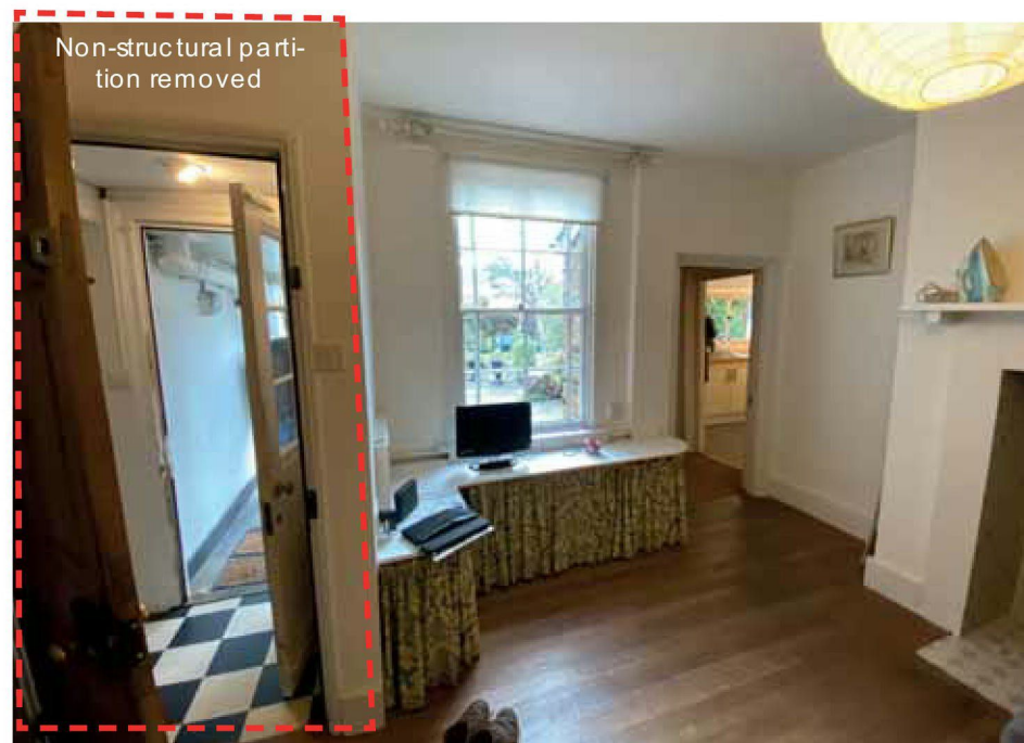
4. Internal Partition removed
