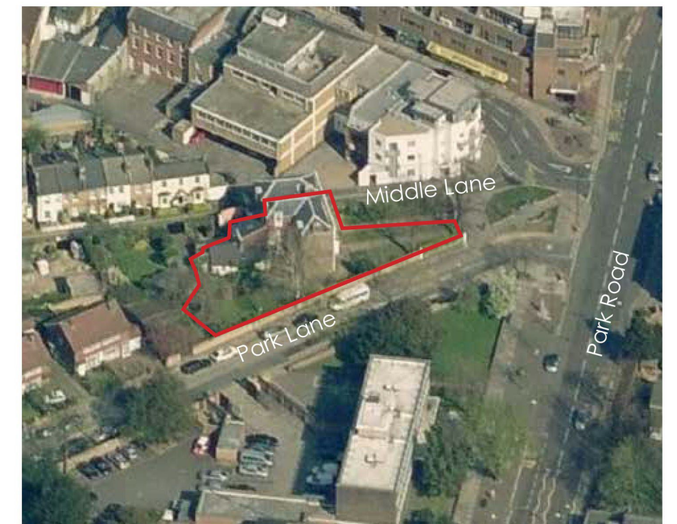
Aerial View of Site
