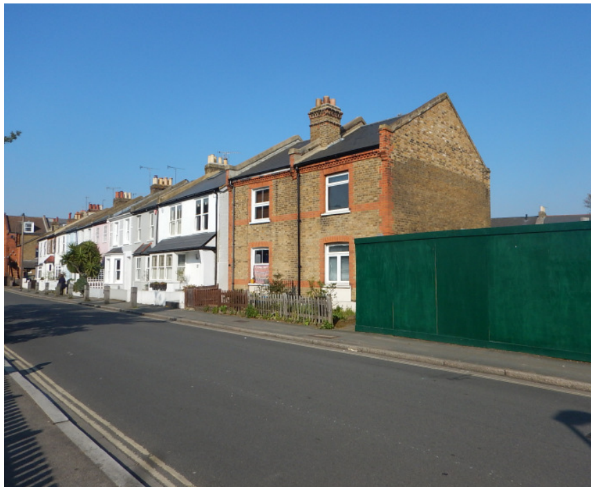
NORTH LANE DEPOT FROM NORTH LANE
