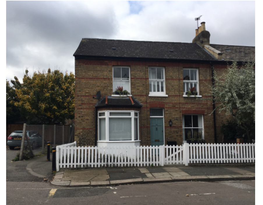
VIEW OF 26 ELLERAY ROAD LOOKING WEST
