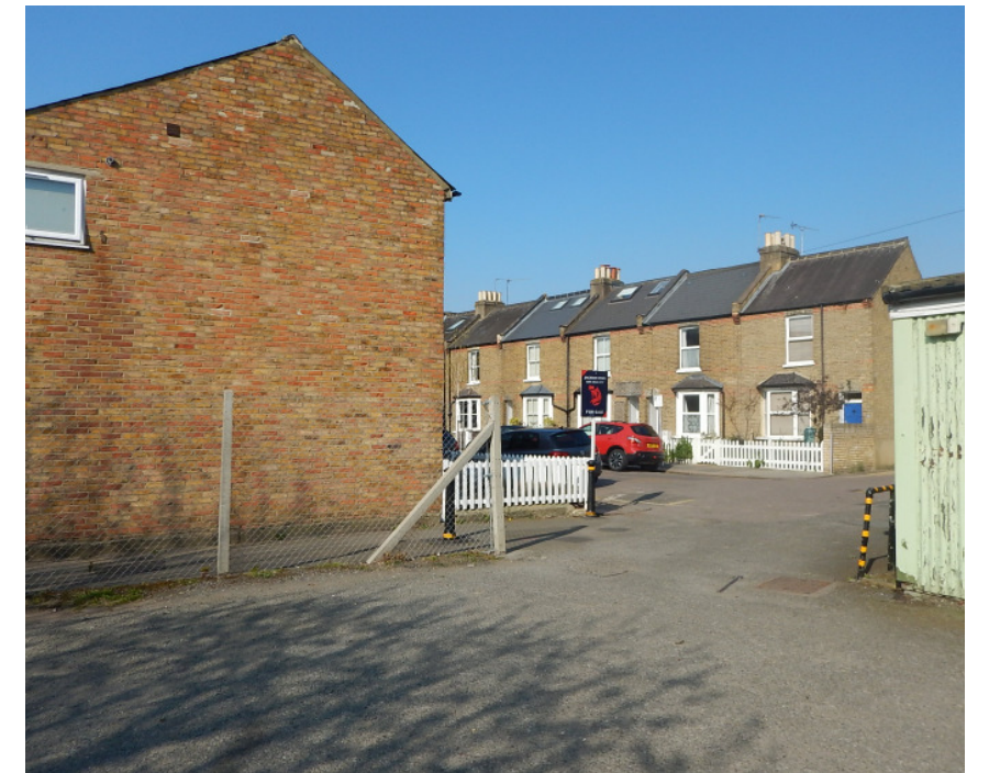
NEIGHBOURING HOUSE FLANK WALL, VIEW FROM CAR PARK
