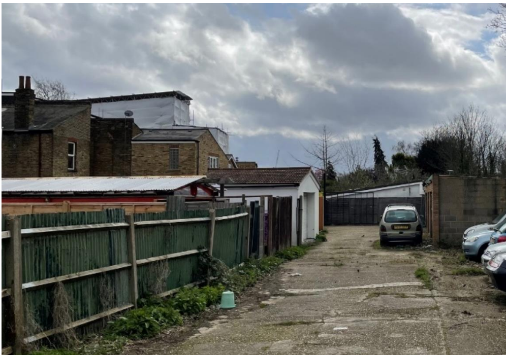
View looking from north to south across the site.
