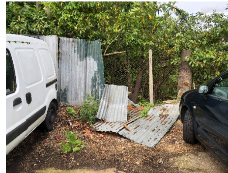
P11: Reptile refugia (damaged section of west boundary corrugated metal fencing)
