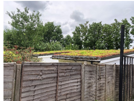
P15: Extensive green roof on building adjacent to south boundary of site
