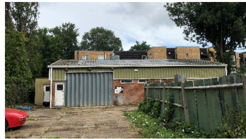
P18: View of south-facing wall of BN1
