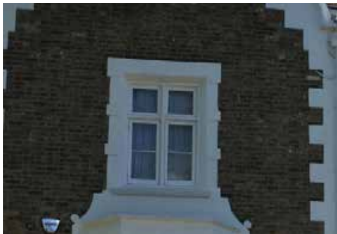
Timber casement with mullion and Queen Anne style transom in a Victorian house
