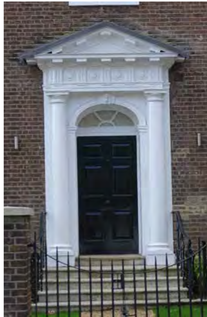
Two-panelled timber door with curved fanlight, classical pilasters and
