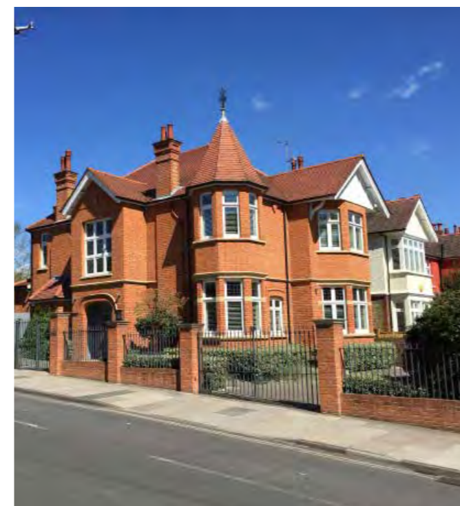
Iron railings, Queen's Road
