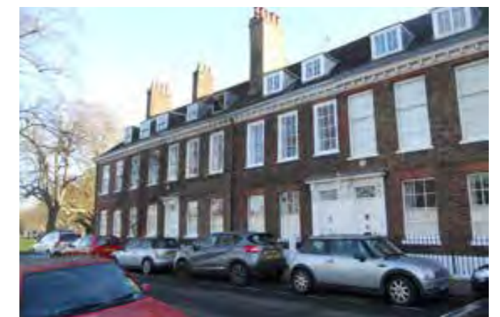
Old Palace Terrace
