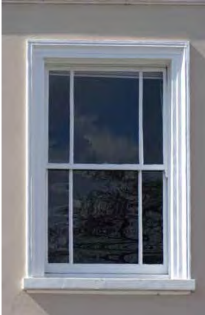
Timber sash with side lights in a Victorian house
