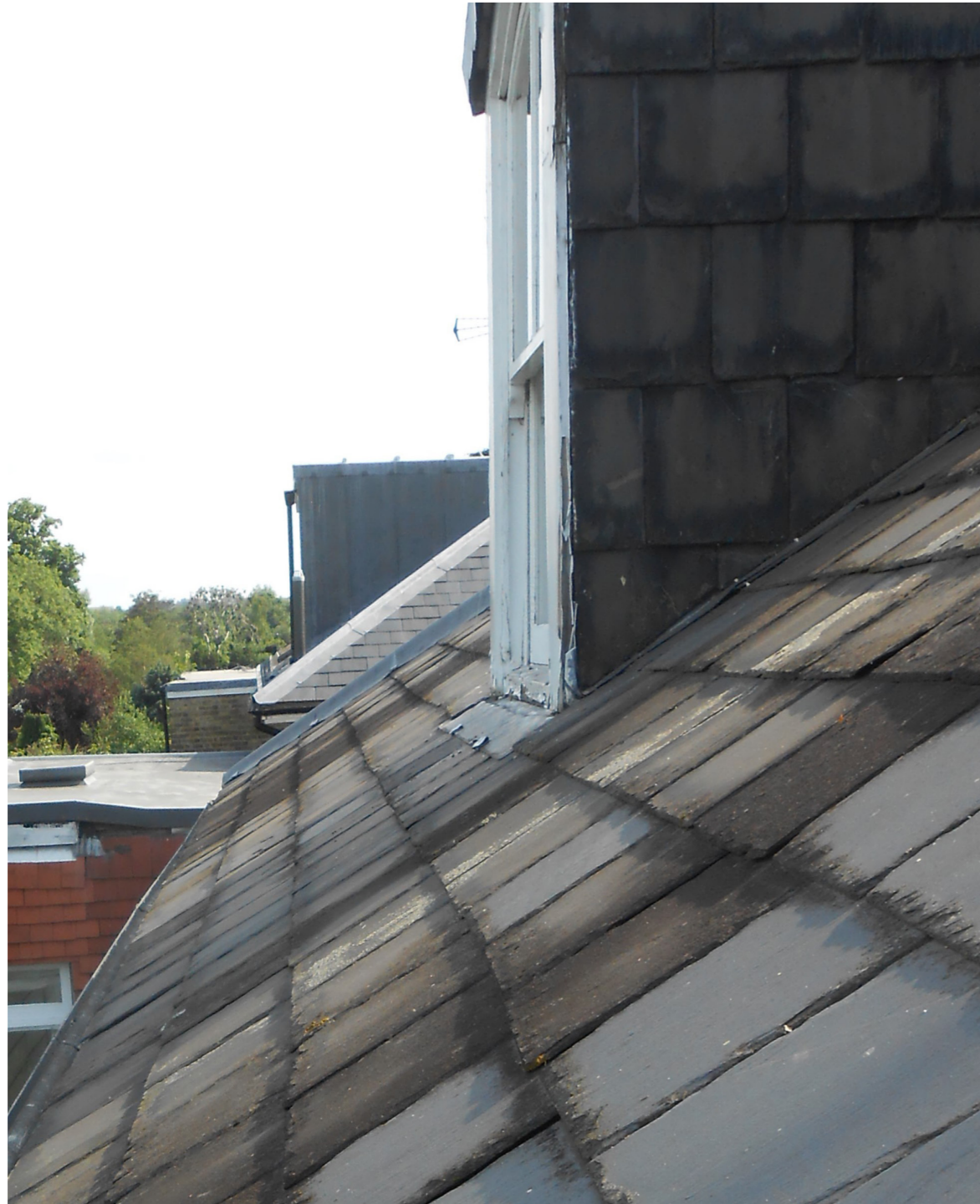
Existing slate roofing (rear slope).
