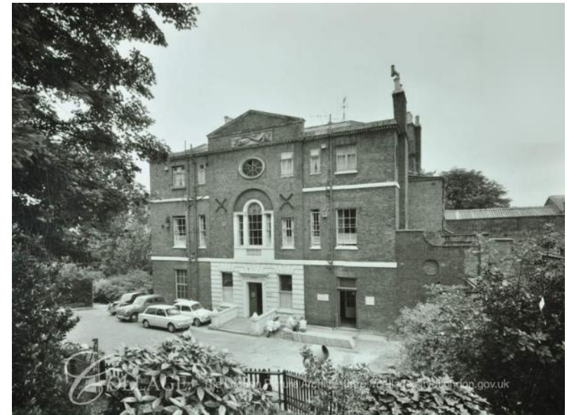
Plate 12: View of the front of Cardigan House from Richmond Hill, 1965 (LMA: 163457).
