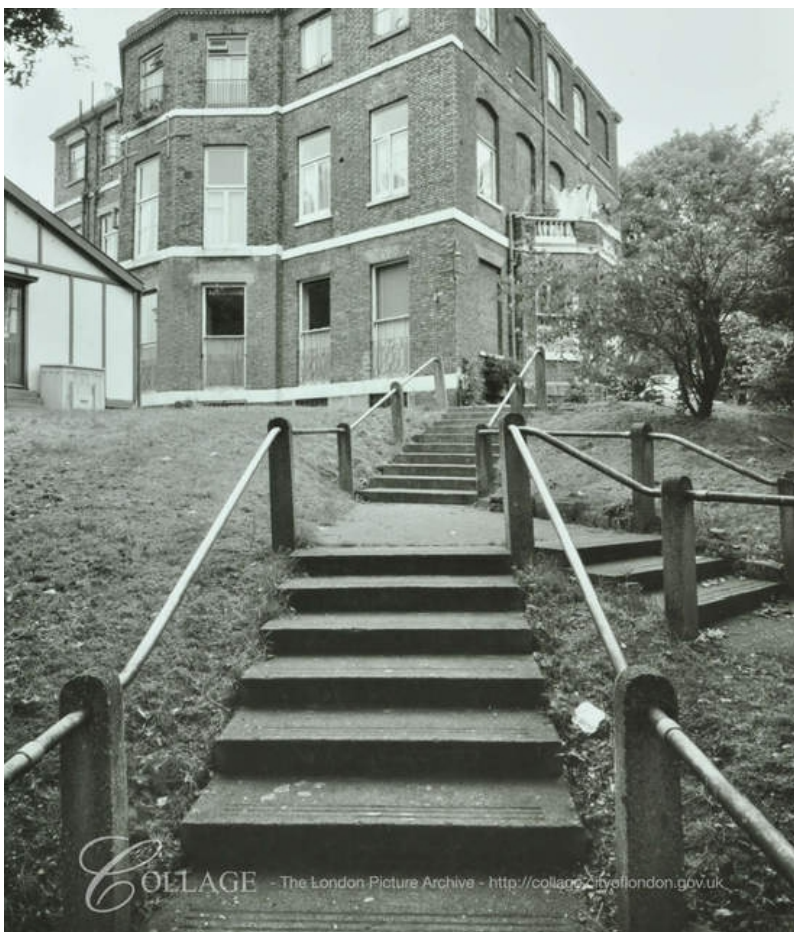
Plate 13: View of the rear of Cardigan House from Richmond Hill, 1965 (LMA: 163445).
