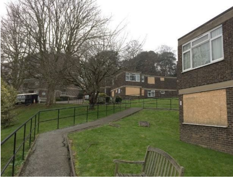
Plate 4: View north from the southern extent of the site
