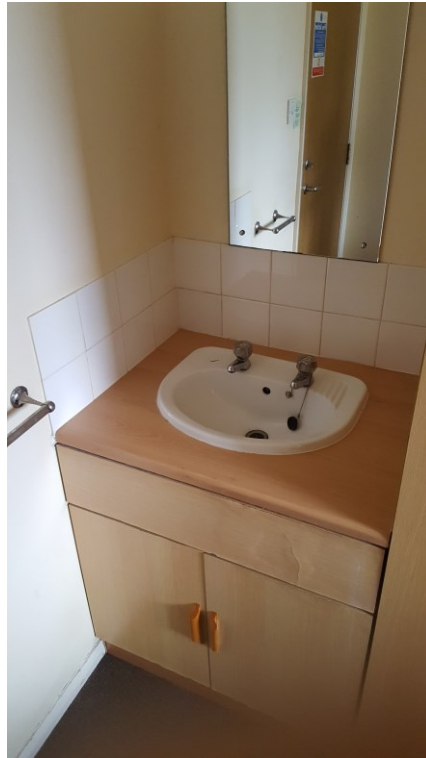
Sink Units to Rooms
