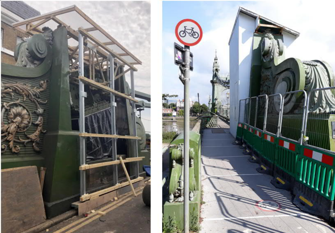
Photo 3.9: Current hoarding around pedestals
