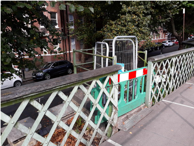
Photo 3.1: Existing opening in parapet for access staircase at the north-west end
