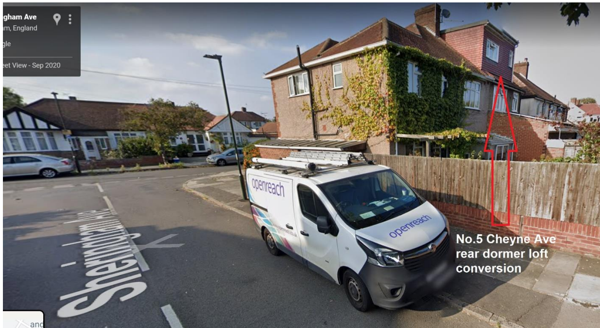
Figure 3. Existing no.5 Cheyne Ave roof rear dormer conversion development
