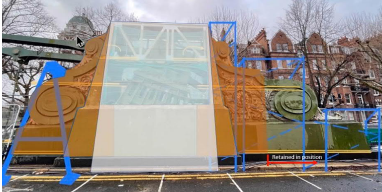
Figure 3.12: Further cast iron cladding panels to be temporarily removed for each pedestal (in orange) to allow access to implement the works
