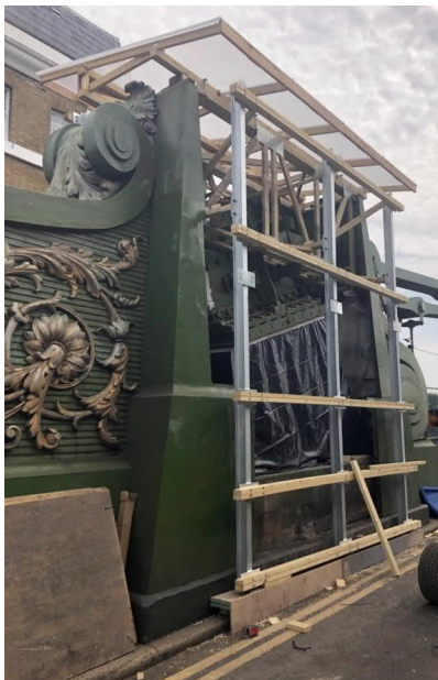
Figure 3.13: Panels removed as described in the 2019 Listed Building Consent application
