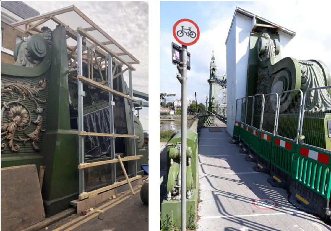
Photo 3.9: Current hoarding around pedestals
