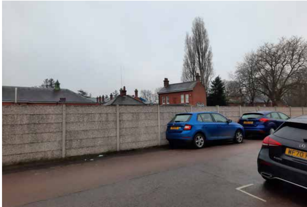
Figure 6.10 Photograph of the Entrance Lodge and Gatehouse from the east on North Worple Way. Photography taken in winter 2021.
