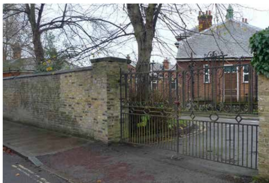
Figure 3.23 The wrought iron gates of the original hospital entrance.
