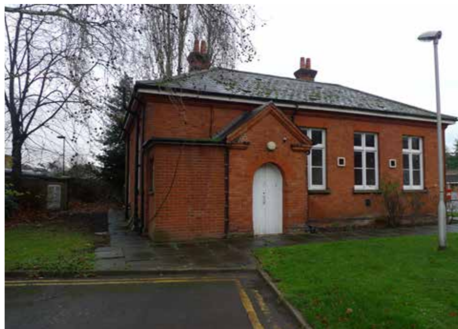
Figure 3.18 West elevation of the Recreation Hall (1903–4).
