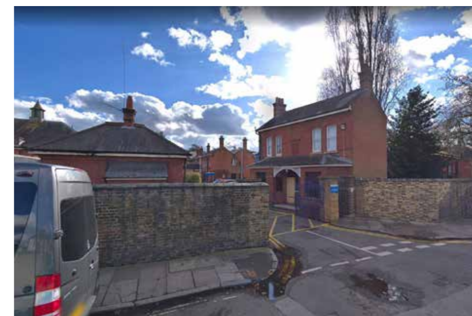
Figure 3.24 The view of the Edwardian BTMs provided by South Worple Street.
