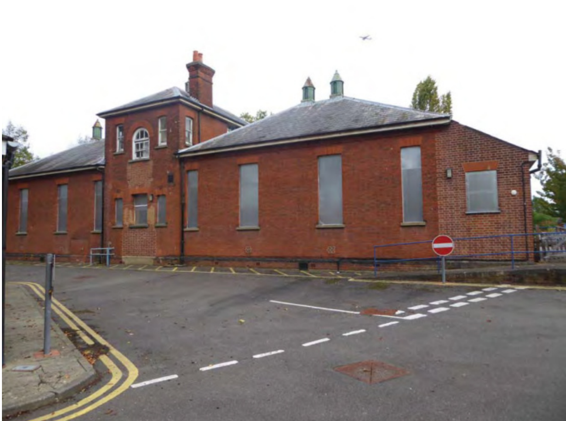
Plate 6: View south west of 1930s building, Barnes Hospital
