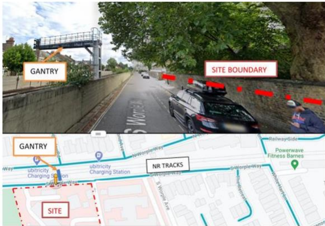
Figure 2-7: Location of Gantry over NR tracks north of site (Source: Google Maps accessed April 2021)
