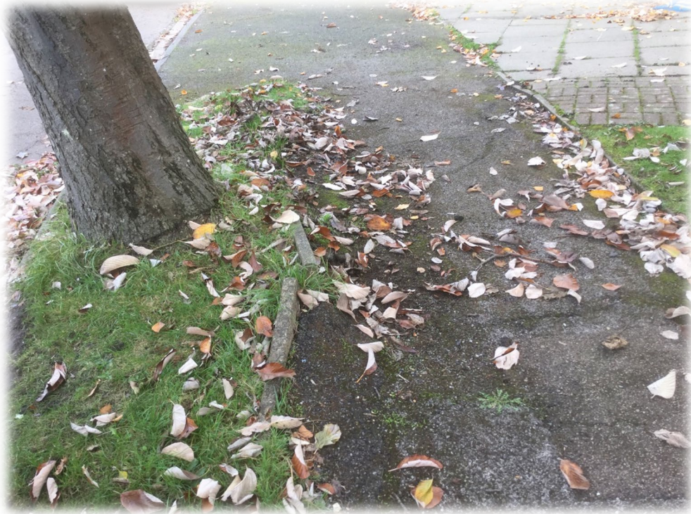
Figure 5: Damage to footpath
