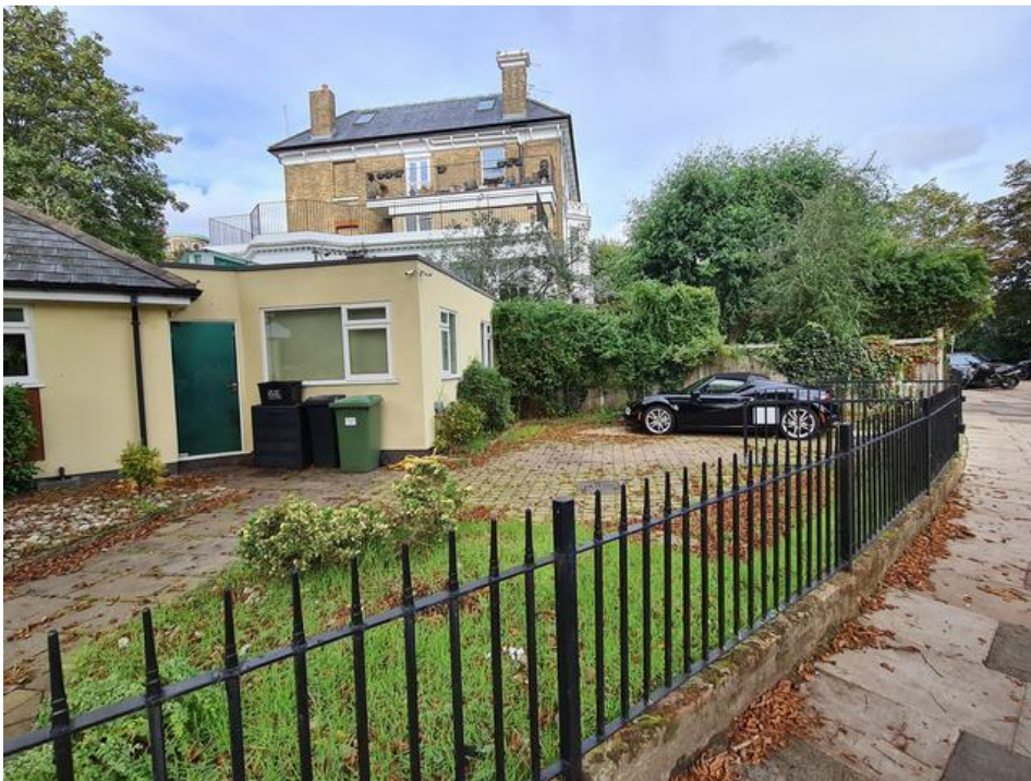
Image 12 Existing entrances and hardstanding areas to the front (south) of the property.
