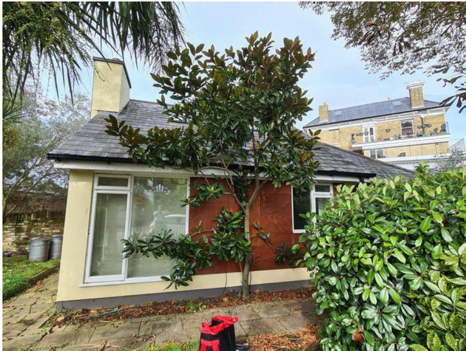
Image 6 T02 growing against the front of the building, to be removed for site access.
