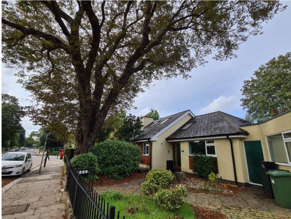
Image 3 Lower crown of T01 well clear of the existing building.
