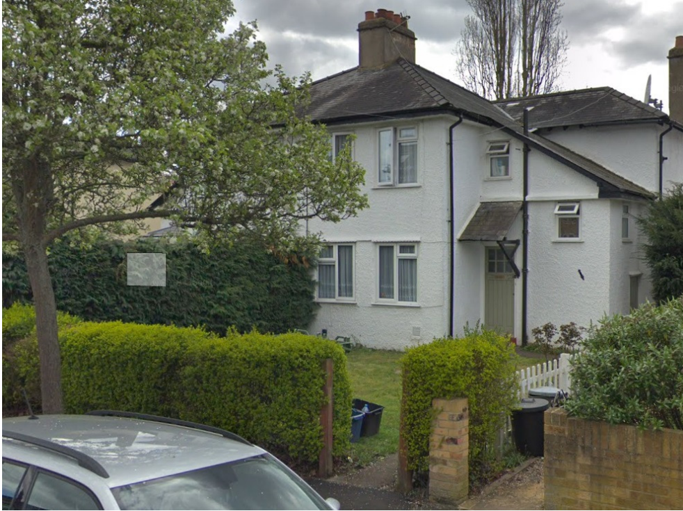
No.31 Kings Road, pre-works (Google Streetview, April 2018)
