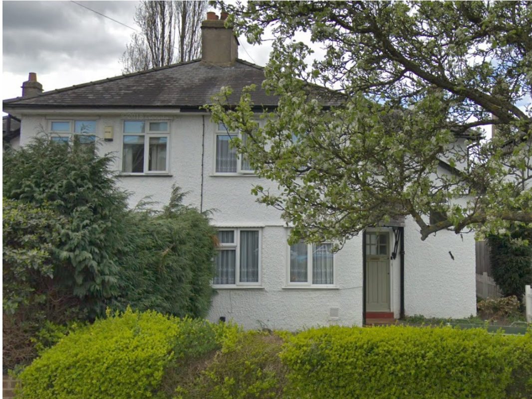
No.31 Kings Road, pre-works (Google Streetview, April 2018)
