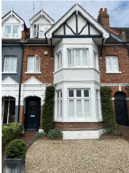
Image 1 - View at No.12 Gloucester Road
