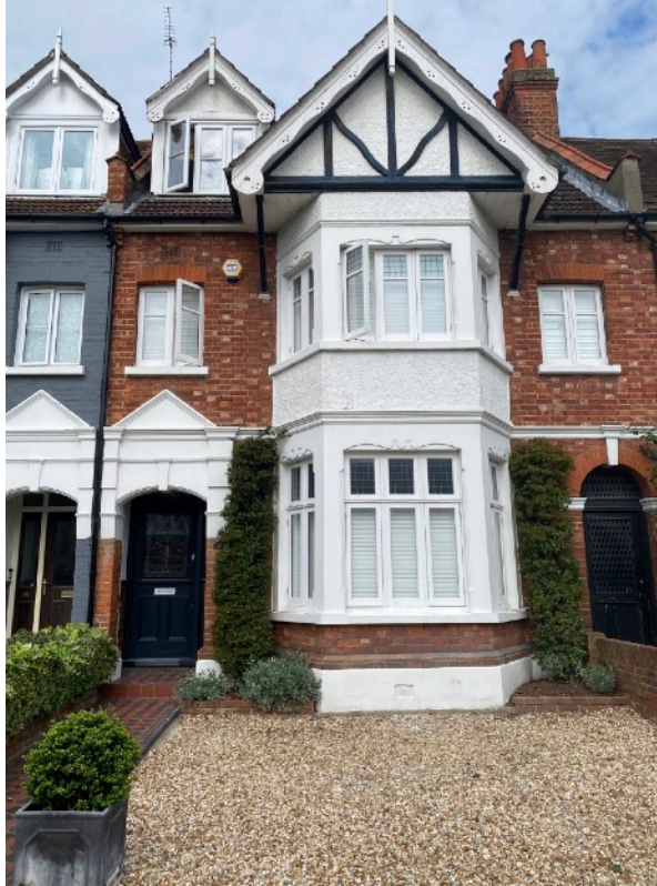
Street view showing No.12 Gloucester Road
