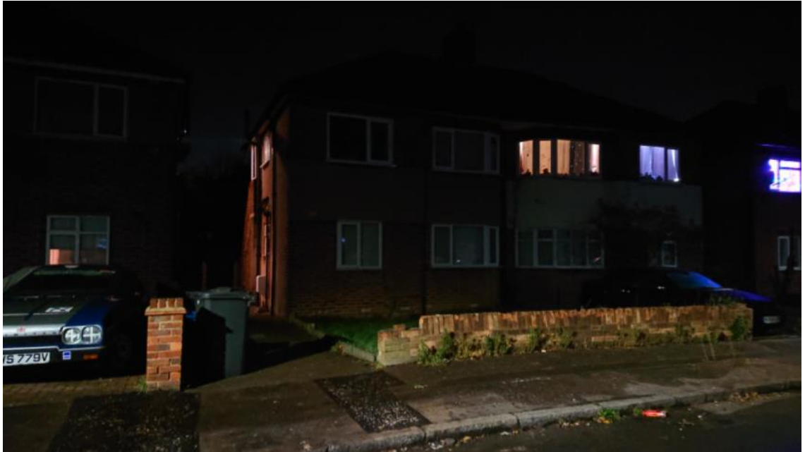
Figure 4.2: Street Frontage Picture of 37 Redfern Avenue, Whitton, Hounslow
