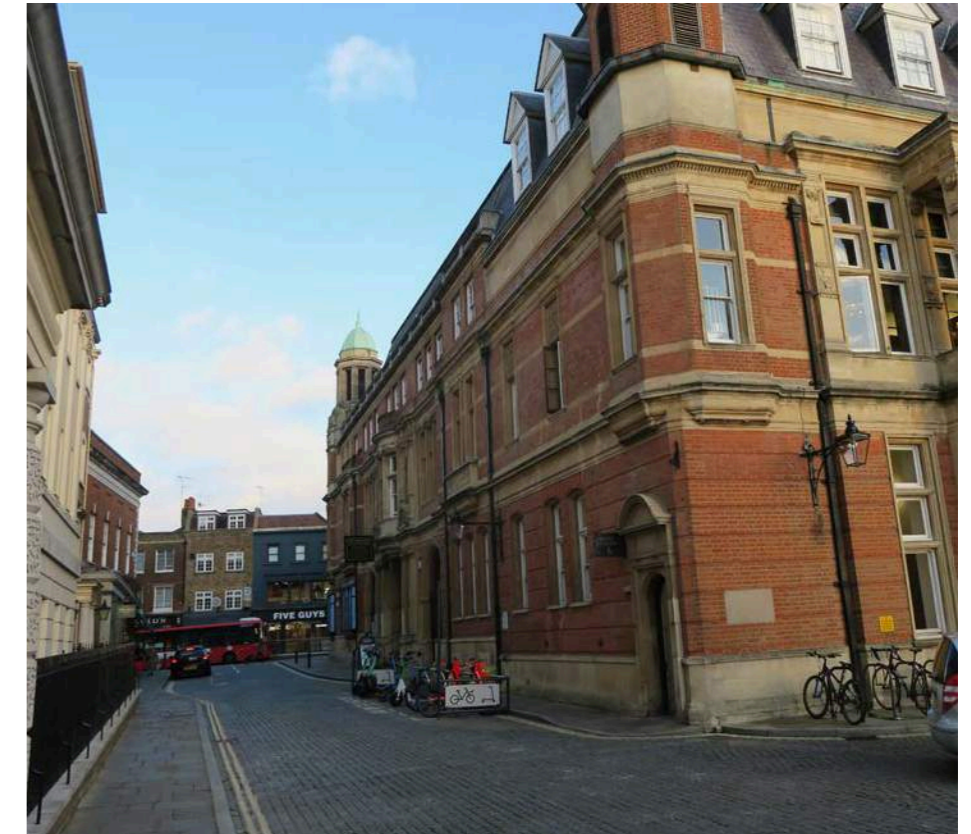
Figure 4.14 Former Town Hall, facade to Whittaker Street and the rear courtyard.
