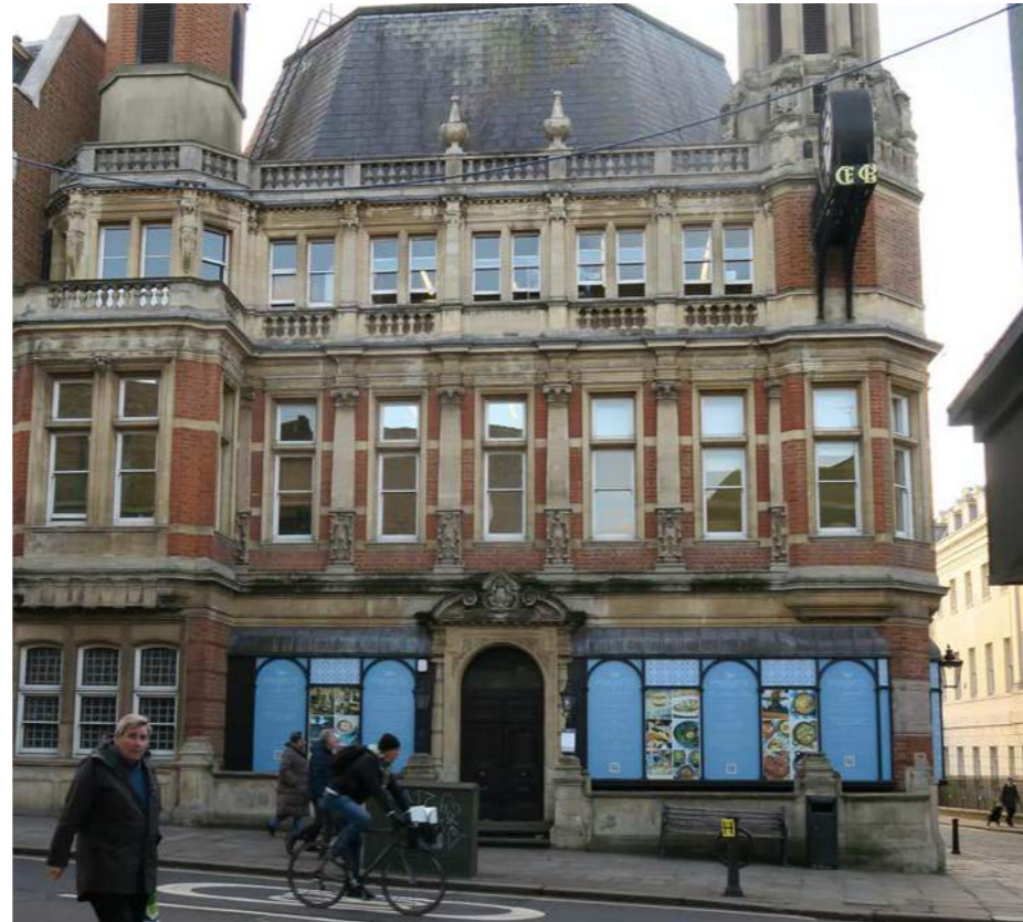
Figure 4.13 Former Town Hall, Hill Street facade
