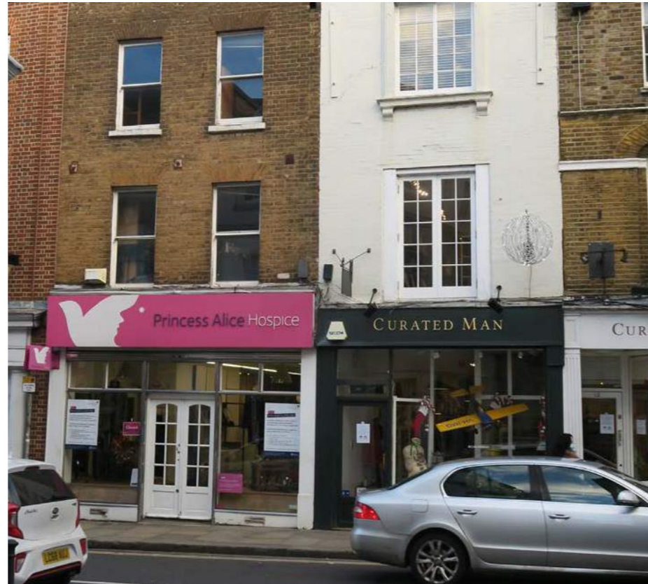
Figure 4.7 Nos. 8 & 10 Hill Street.
