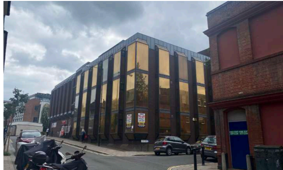
1. View from Lewis Road
