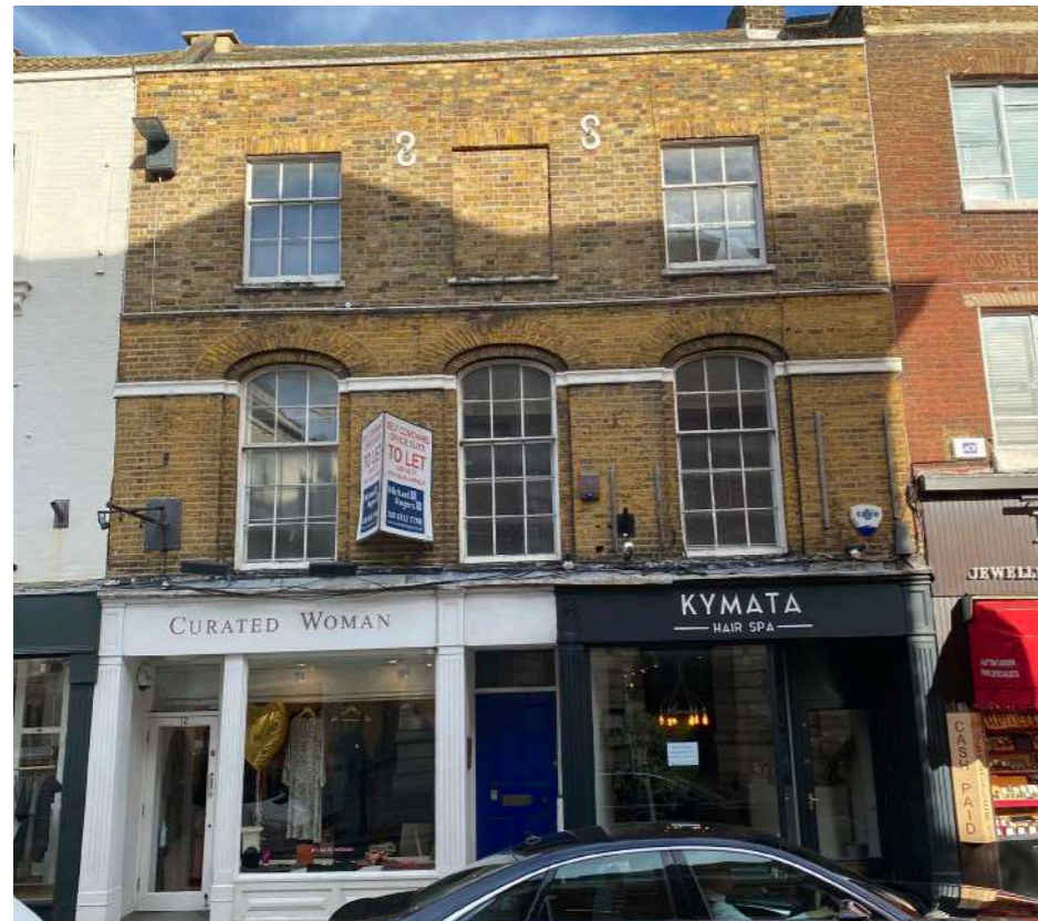
3. 12 & 14 Hill Street, Grade II listed building
