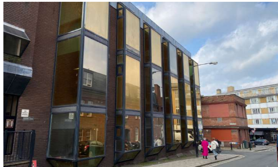
3. View from Lewis Road
