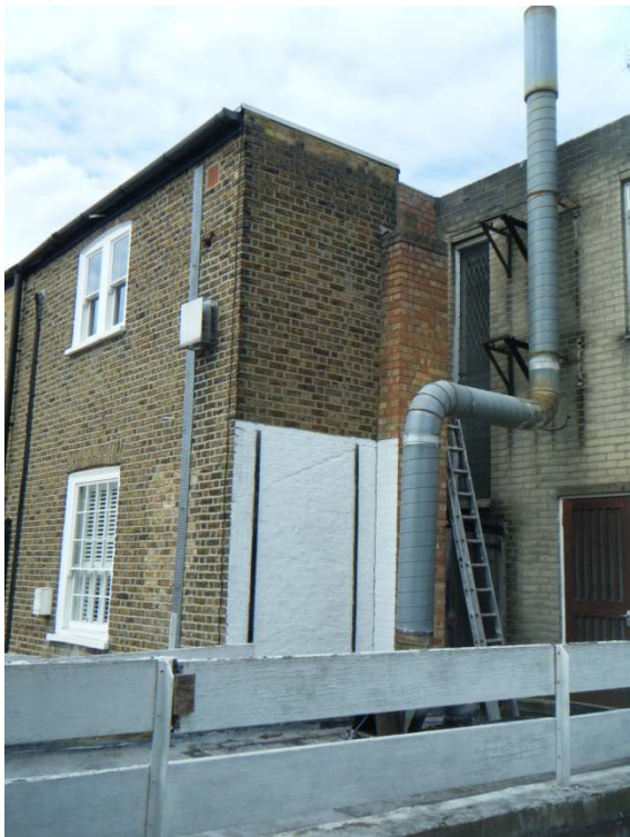
REAR OF No. 12 KING STREET
