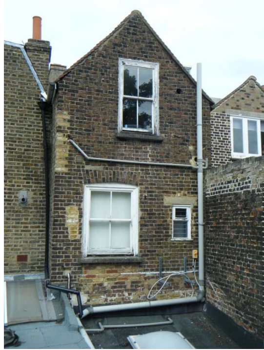
REAR OF No. 9 KING STREET
