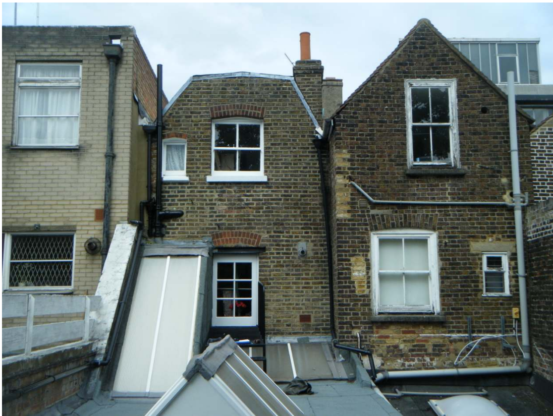
REAR OF No. 10 KING STREET
