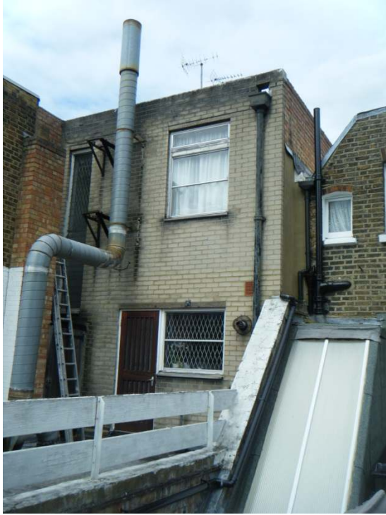
REAR OF No. 11 KING STREET
