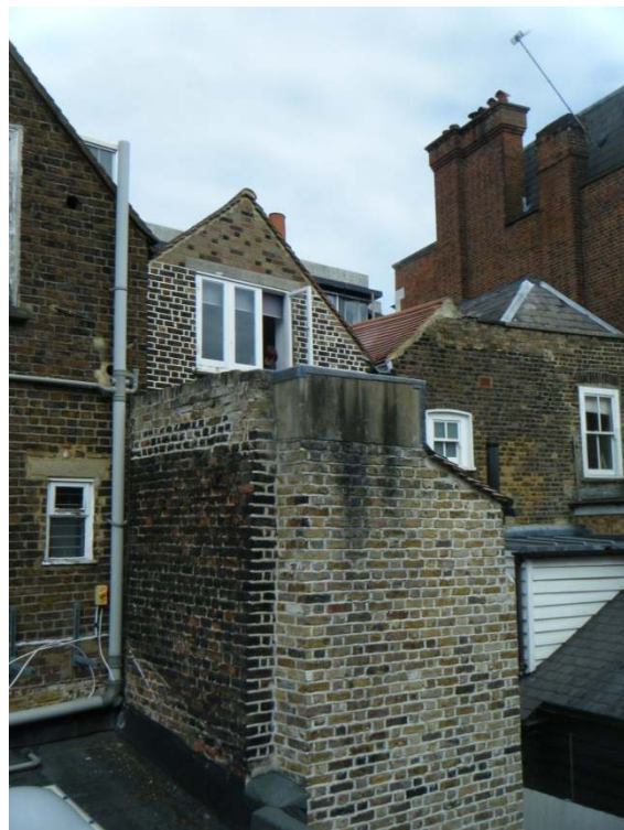
REAR OF No. 8 KING STREET
