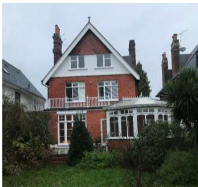
Rear Elevation of 2 Broom Water West
