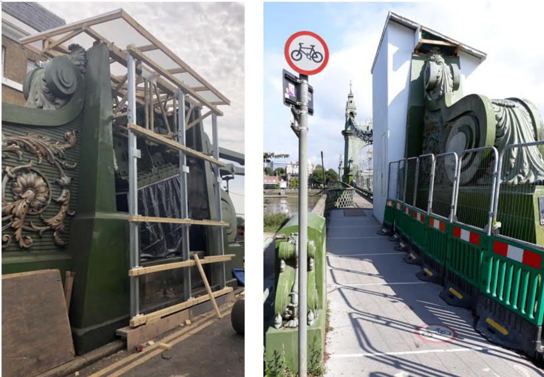
Photo 3.9: Current hoarding around pedestals
