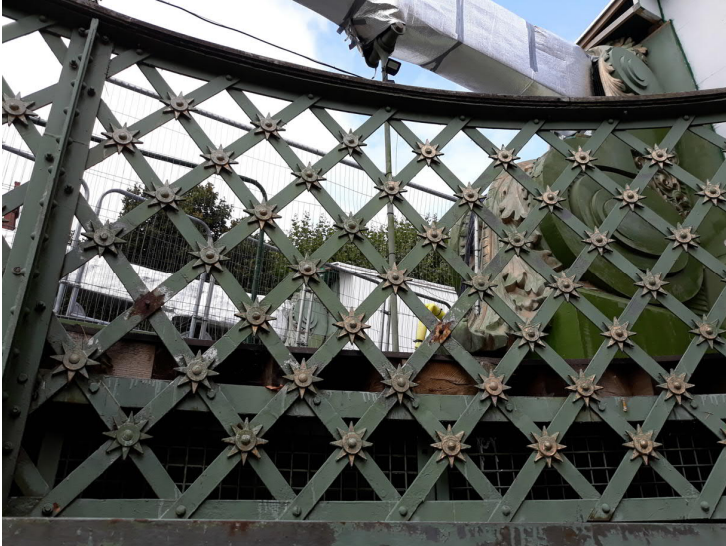
Photo 3.2: Typical parapet near north-east pedestal, viewed from adjacent ramp
