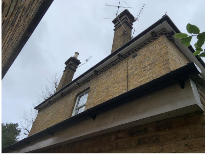
Photograph 4 Southern elevation of B1.2 and B1.8.
