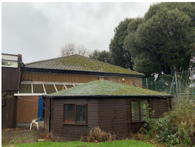
Photograph 3 Building 2 southern elevation And Building 1 section B1.4 southern elevation
