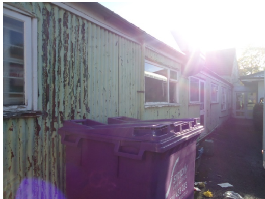
Extension to west side, with later extension beyond
