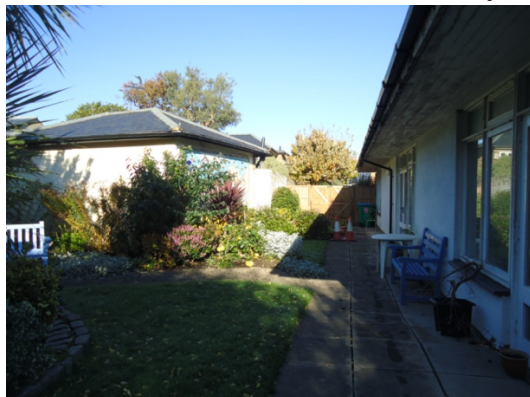
Extension to rear - west
