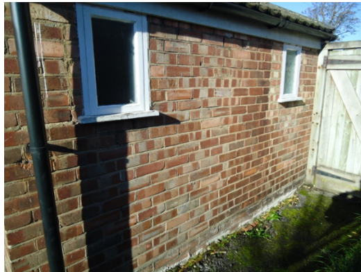
Brick extension to the front (east side)
