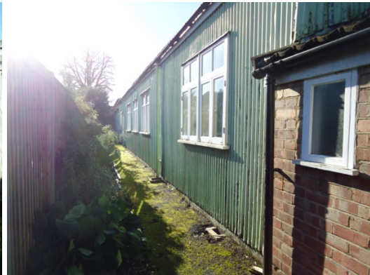
Plain and undetailed east elevation of main building
