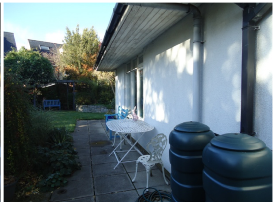
Extension to rear - south
