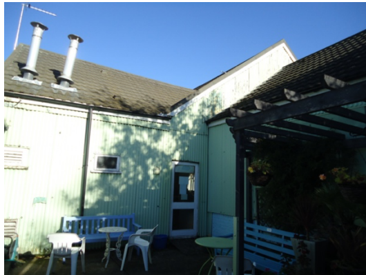
View of rear of main building
