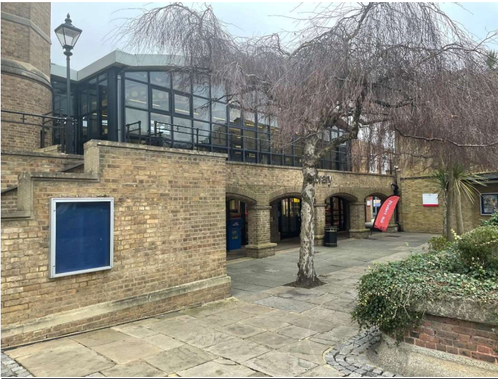
Existing Guardrails above Library
